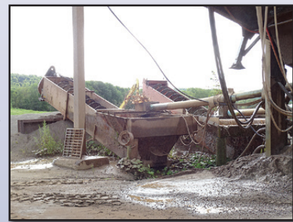
HYDRAULIC WASH PLANT
