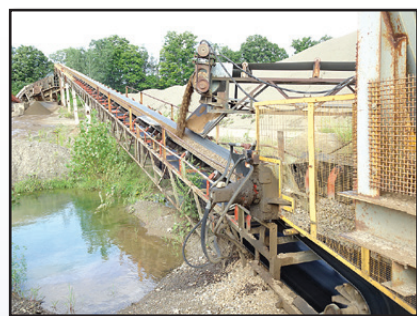
HYDRAULIC WASH PLANT
